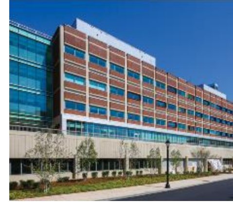
Gant Building Renovation Phase I-II
